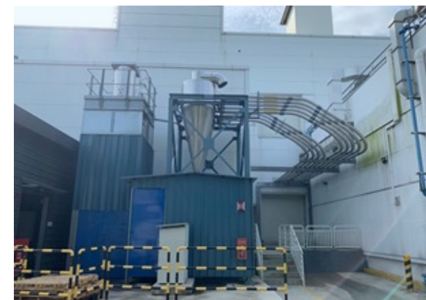
THE POLYPROPYLENE MOLD WASTE COLLECTION SYSTEM SILO IN SINGAPORE
